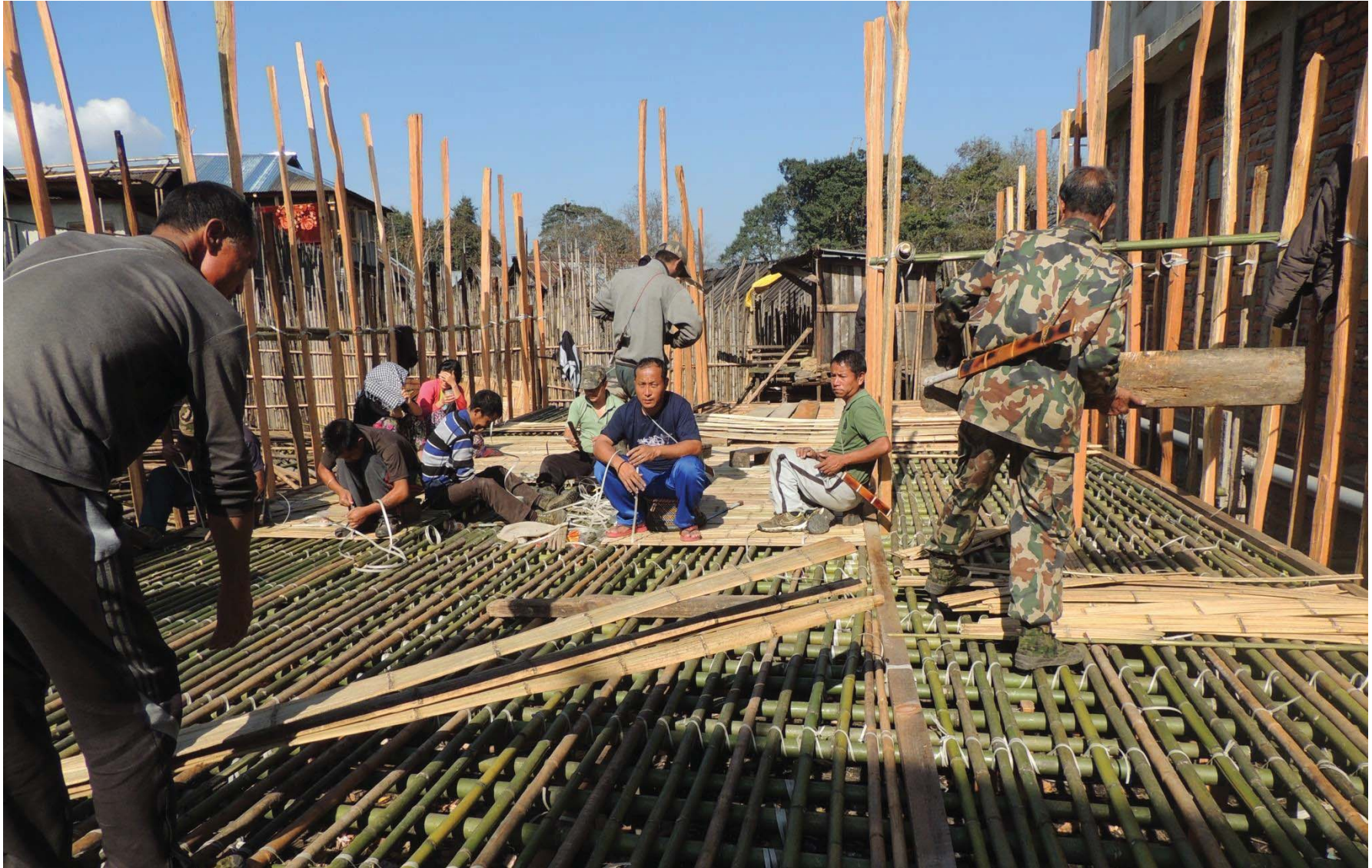
Members of the basti get together and repair a house, Hong village
