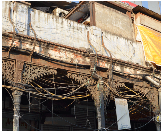
Dilapidated buildings of Chandni Chowk.
