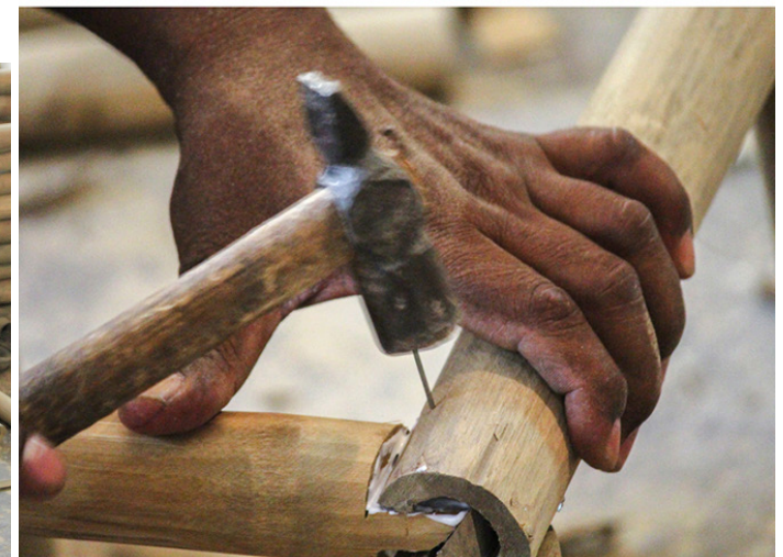
Nail is fixed near the joints of bamboo to hold it strong.
