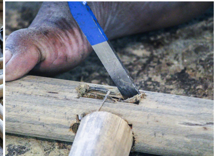
The holes are opened bigger to attach another piece of bamboo.
