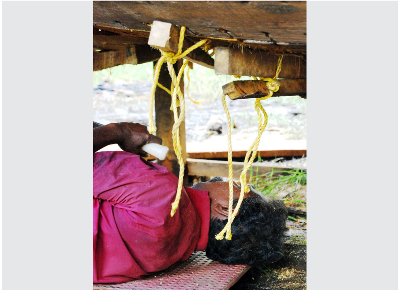
The raised platform enables easy accessibility for the craftsmen to construct the boat.
