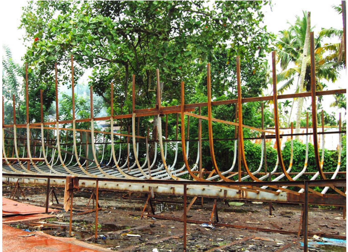
The metal skeleton structure of the keel and the ribs.
