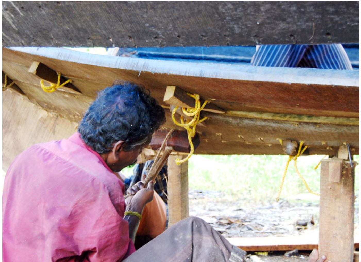
The coir is pulled and tightened using the hammer.
