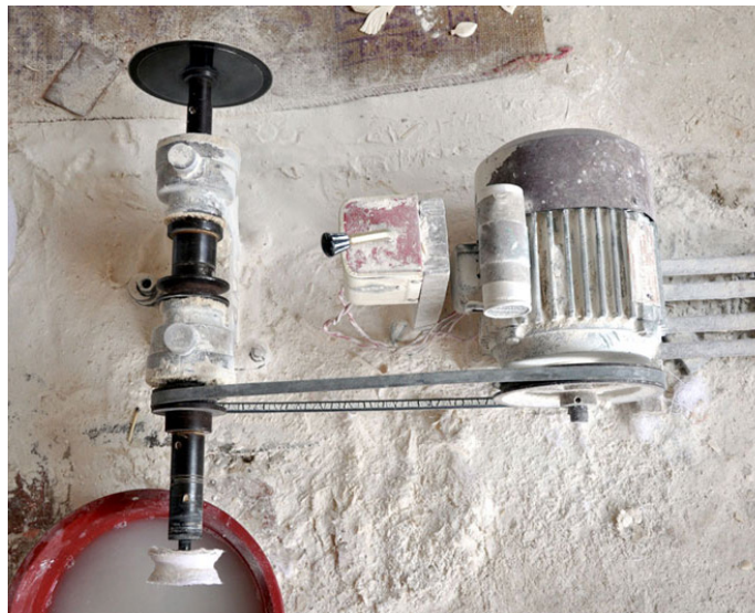
Over-view of buffing machine.
