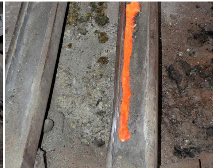
Molten metal being poured in the mould
