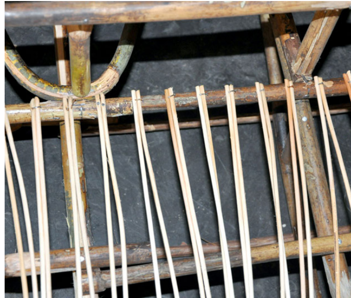
Cane joined to the bamboo with thin small nails.
