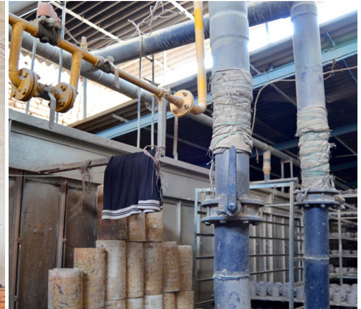
Diesel fired furnace.
