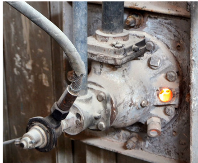
Diesel fired furnace.
