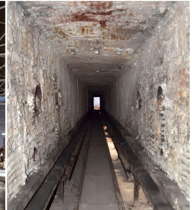
The inside of the furnace (minus the container cars).
