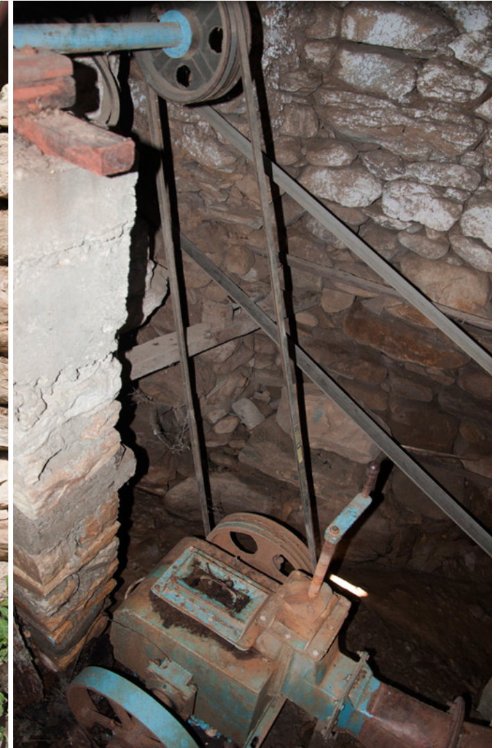
Water force controller junction.
