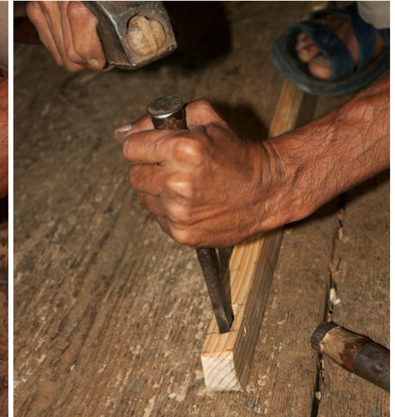
Holes are made using chisels and hammer to insert the other parts to be fixed together.
