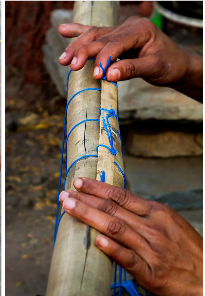
Guides are suspended at equidistant and strips are fasten.
