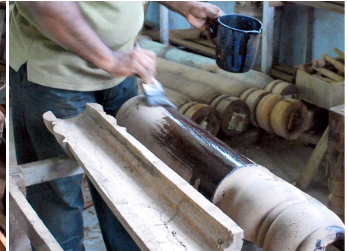
Chemical pesticide is applied on the outer surface of the pillar to keep termites away.
