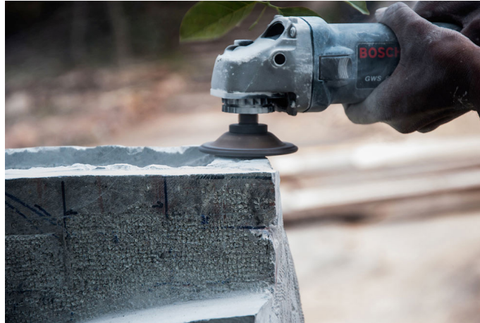
Buffing machine is used to smoothen the stone.
