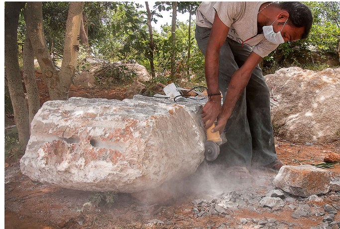
Roughly cutting the rock with the help of stone cutting machine/angle grinding machine.
