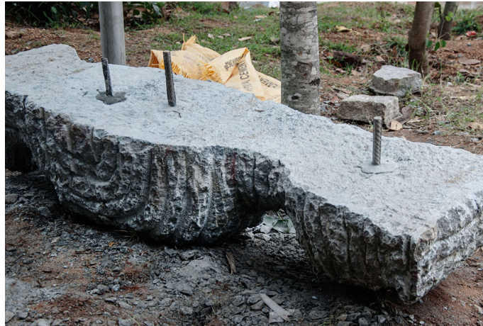
Iron rods are placed in the drilled holes.
