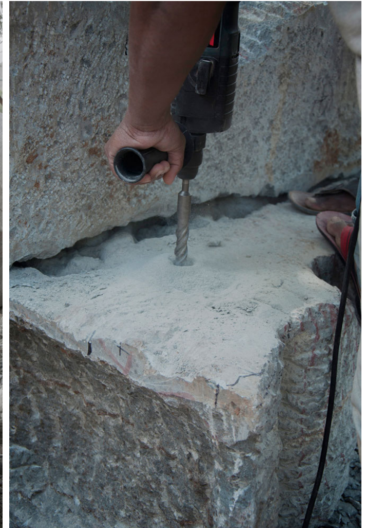
Drilling the marked holes.
