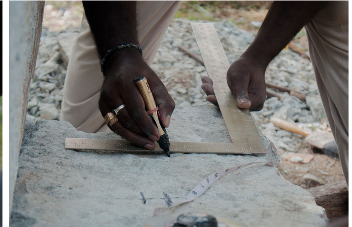
L shaped square tool is used to mark on the stone.
