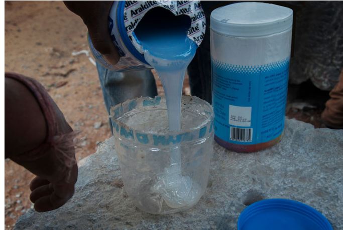
Epoxy resin (Araldite) is poured.
