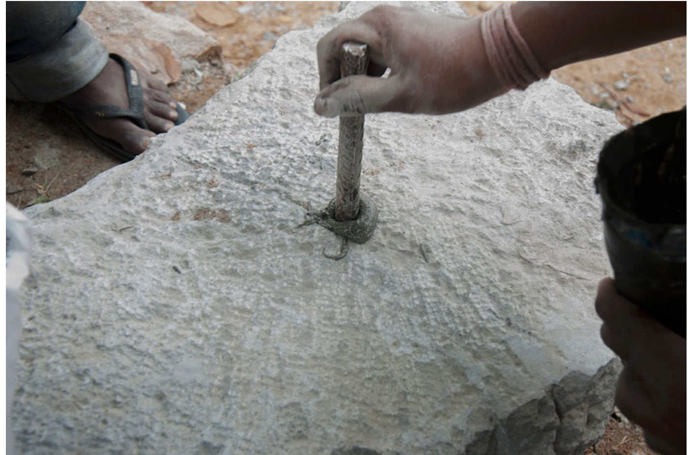
Iron rod is placed into the hole.
