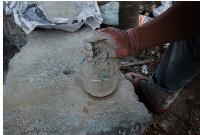
Stone powder is mixed with the resin.
