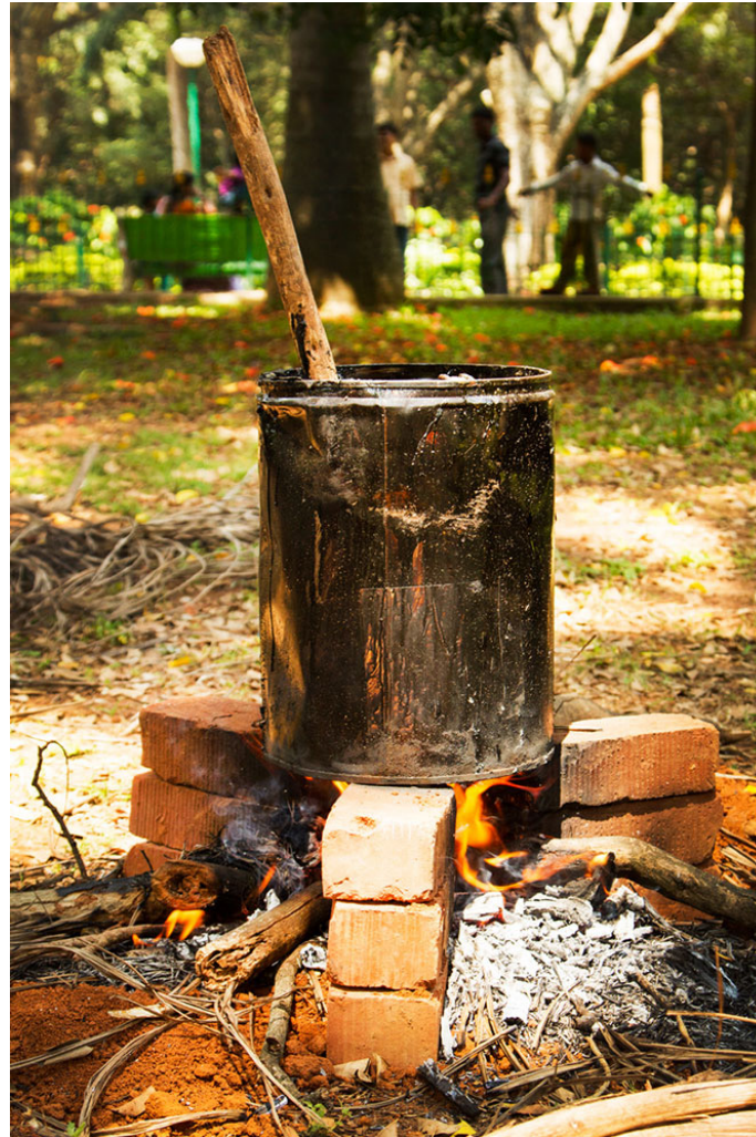
Tar is used in installing the work.
