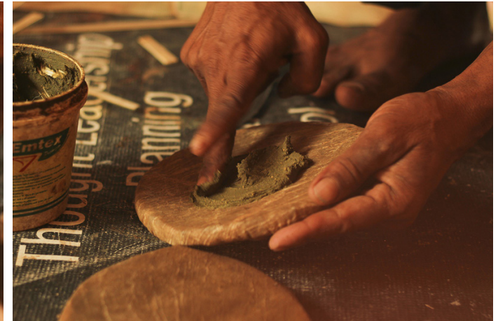
A mixture prepared of Sahi Kare, grease, lime stone solution and used engine oil is applied on the membrane.
