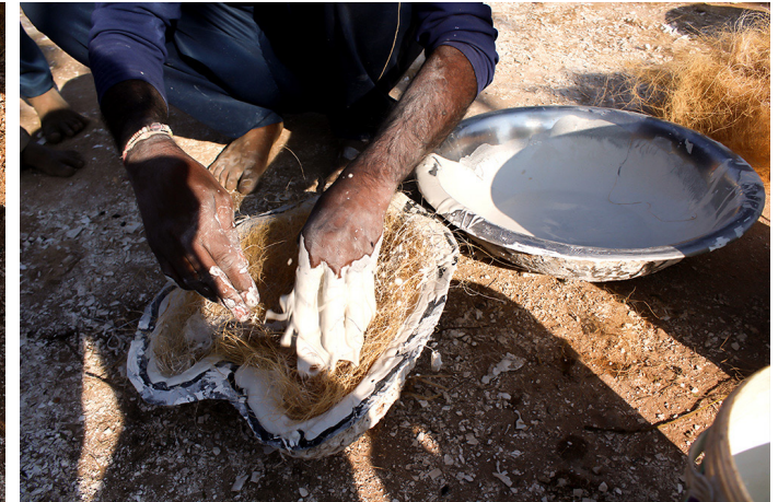
Again giving another layer of POP liquid on the coir.
