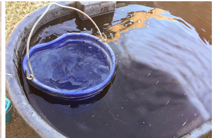
Water is used to mix the powder of plaster of paris in thick density.
