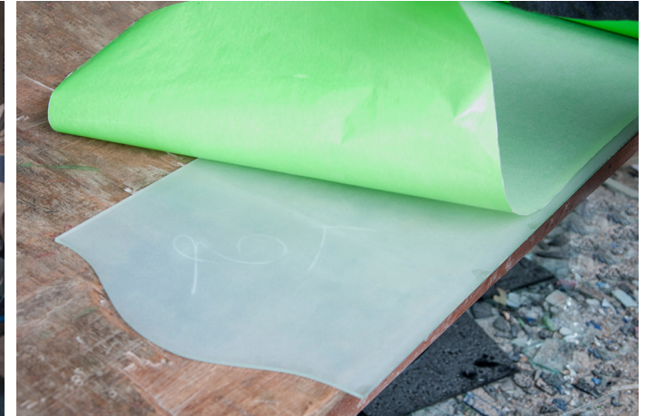
Vinyl sticker sheet is spread on the glass slab.
