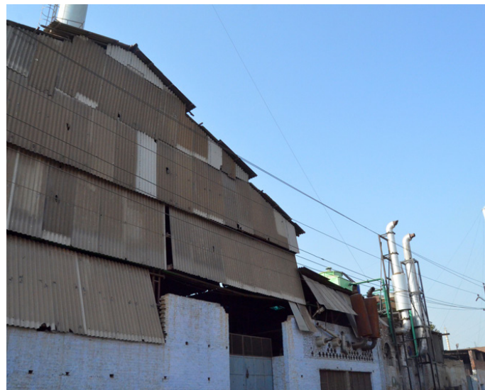
Firozabad industrial area.
