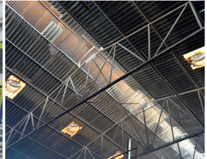
The exhaust fans in the factory.
