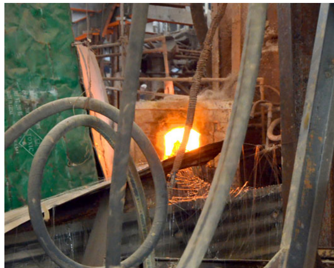
Pipelines in the factory.
