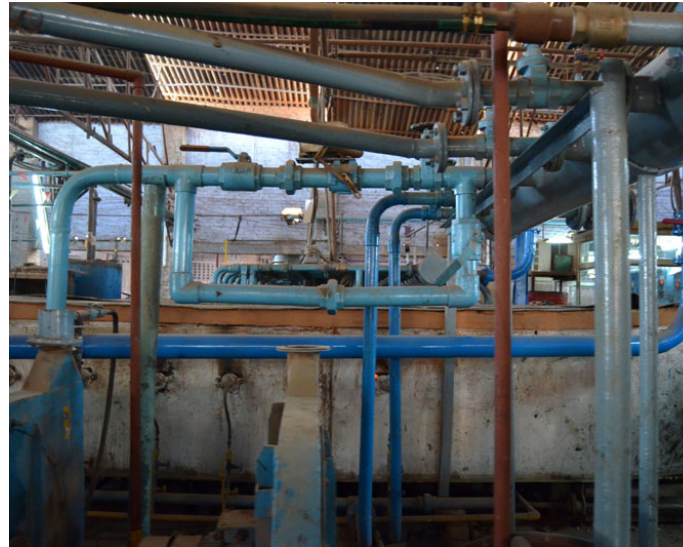
Pipelines in the factory.
