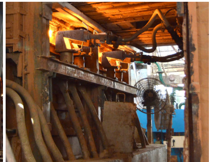
The gas burners of the furnace.
