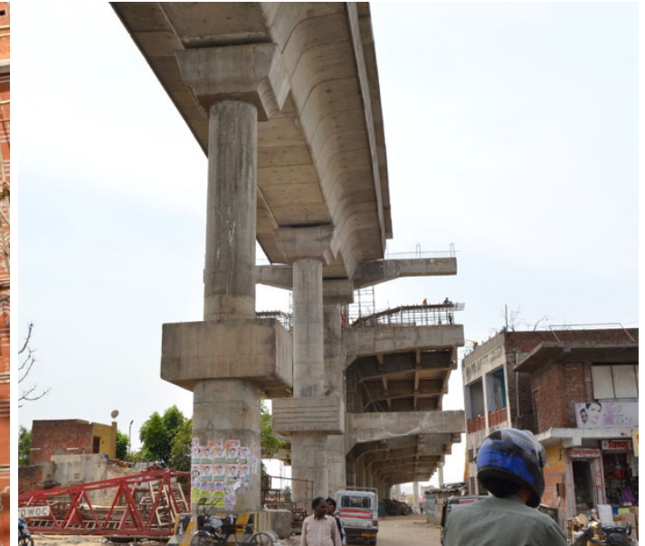
Metro construction in the city.
