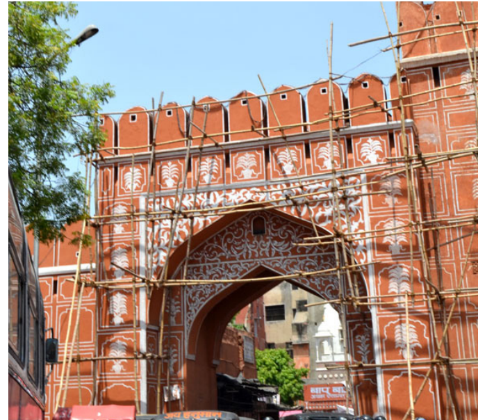
Restoration in progress.
