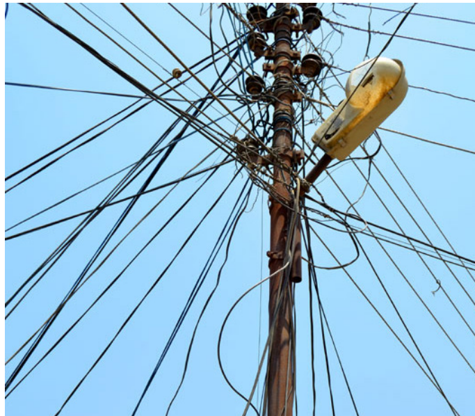
Wired chaos on an electric pole
