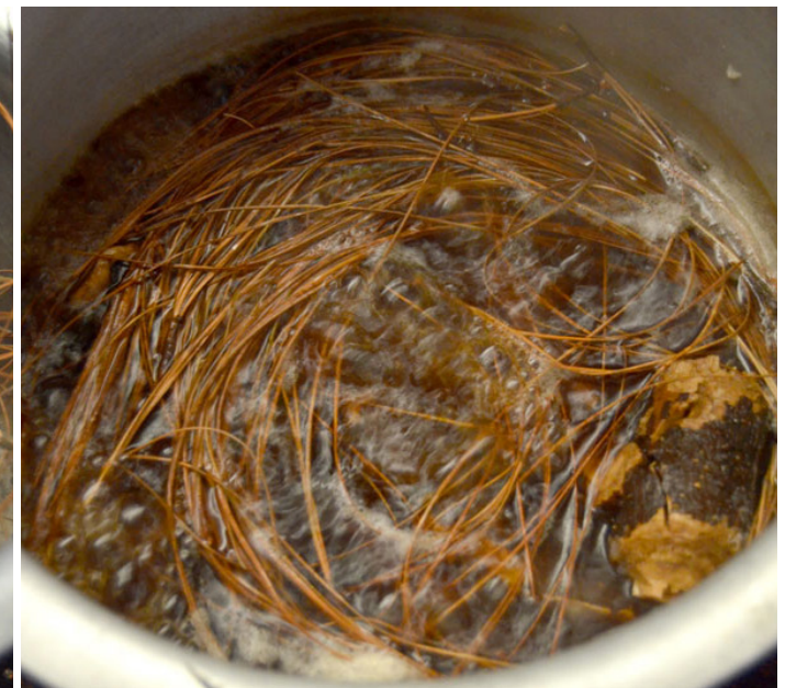
Pine needles being put in the boiler.
