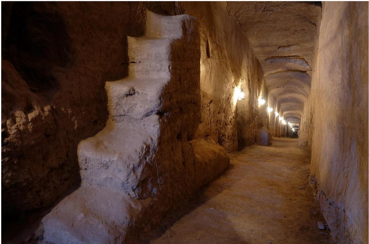
Figure. 9 Hand-dug stairs to the inspection room
