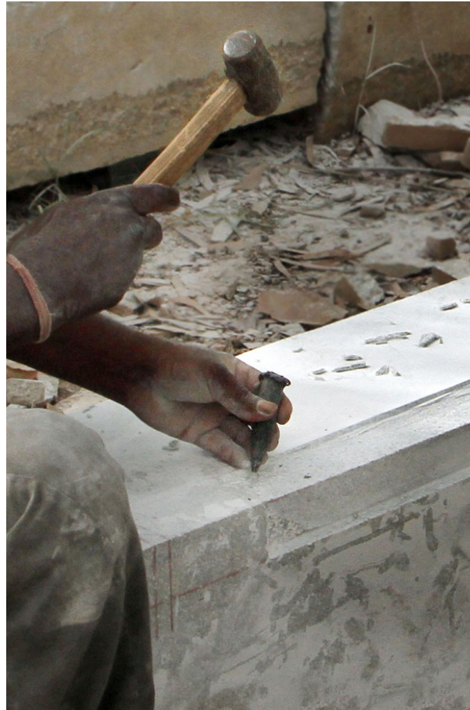
Big chisels are hammered to remove the excess parts of the pillar.
