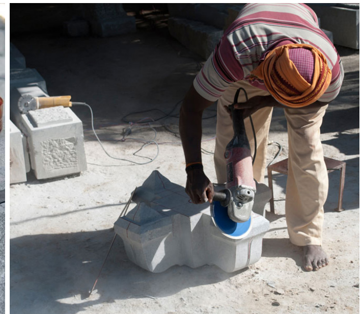
Stone filler, use to make the surface plane.
