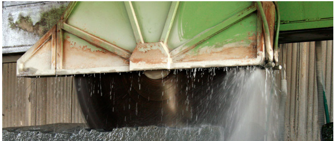
Bigger channel cutter to cut the bigger surface.
