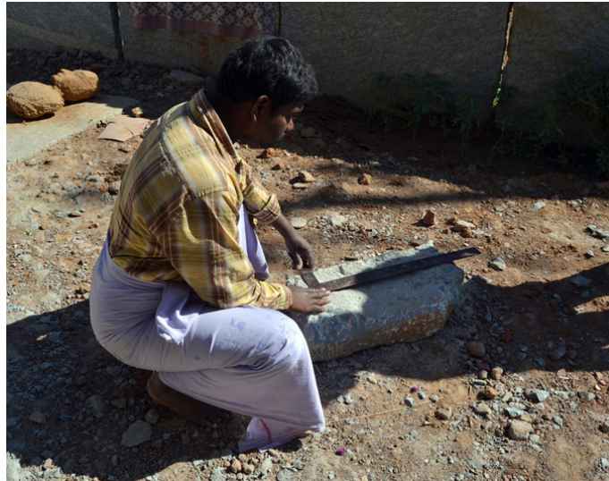
Large scale to mark the stone horizontally.
