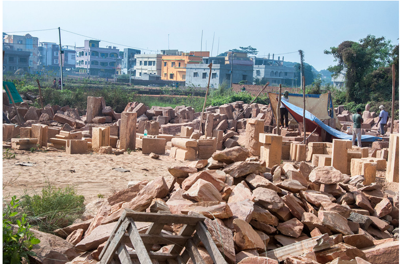
Small and big different stones are set aside in work place.
