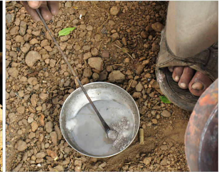
Mixture of eight different metals used to seal the gaps.
