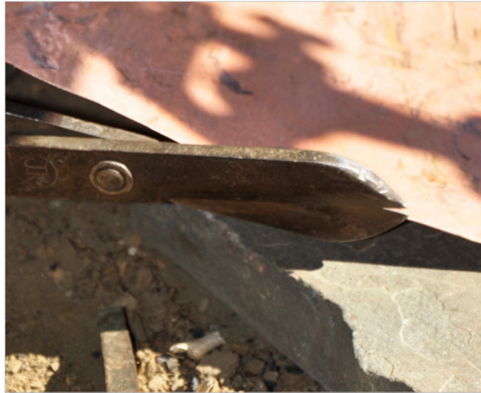
Copper sheet is cut as per required size.
