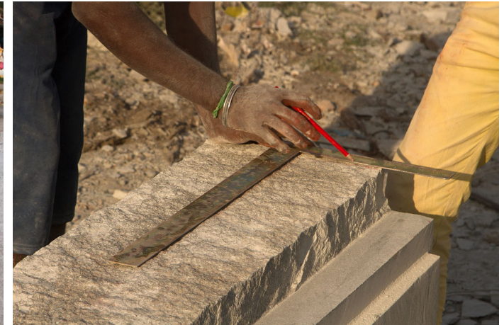
Measurements are marked on stone to cut it to a required shape.
