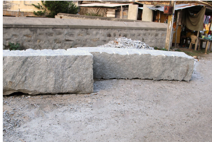
Koira stone cut into huge rectangle blocks to make the pillars for the temple.
