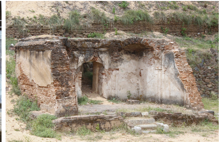
Remains of a building found during excavation.
