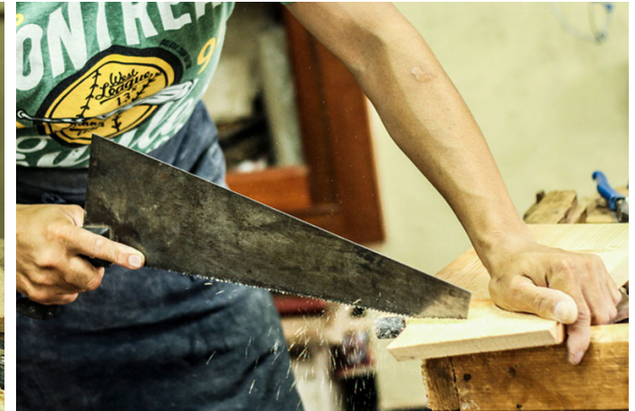
Marked wood is cut with hand saw.
