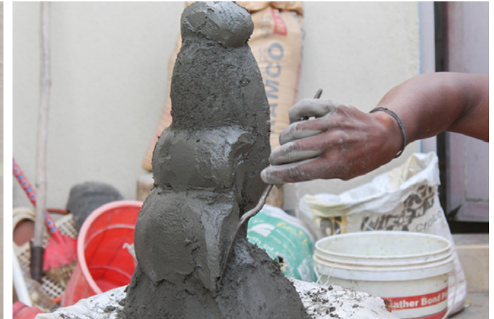
The required shape is achieved by applying soft cement.
