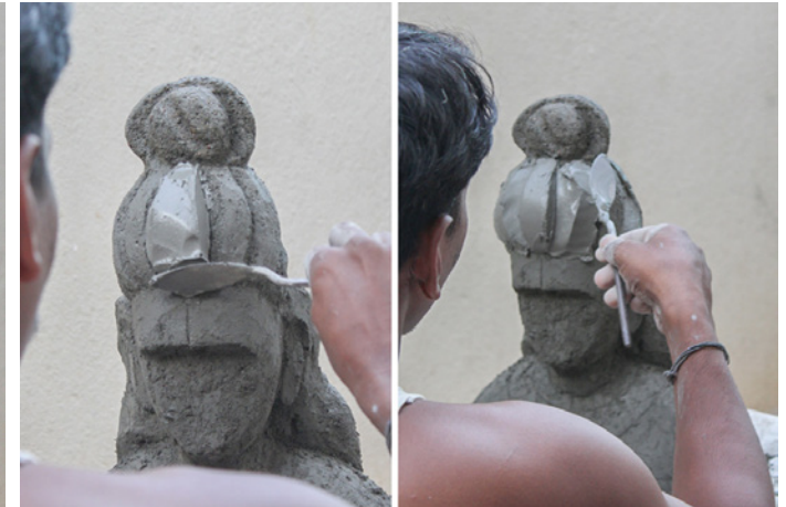
Smooth cement is applied over to give a finishing.
