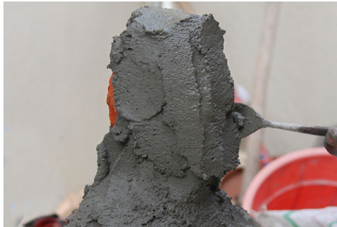
Cement is applied on the brick.
