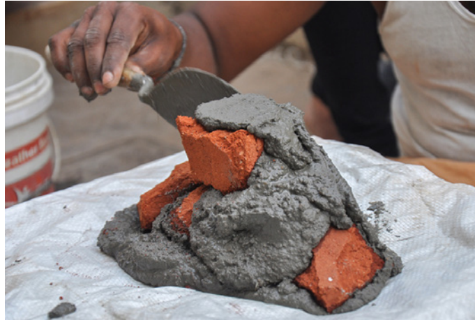
The bricks are packed with cement.
