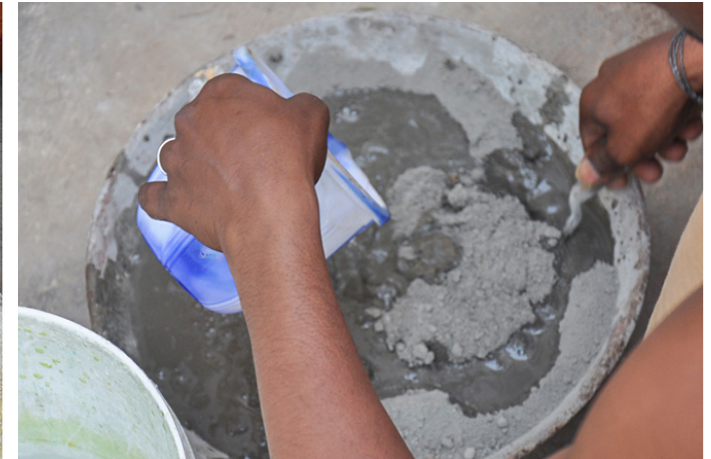
Cement and sand is mixed together with water in right proportion.
