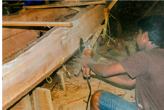
Smoothing the surface with the help of Electric hand buffing machine.
