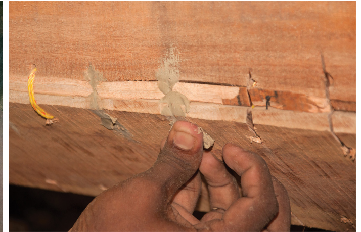
Applying M-seal to fill the line gaps caused by the stitching process.
