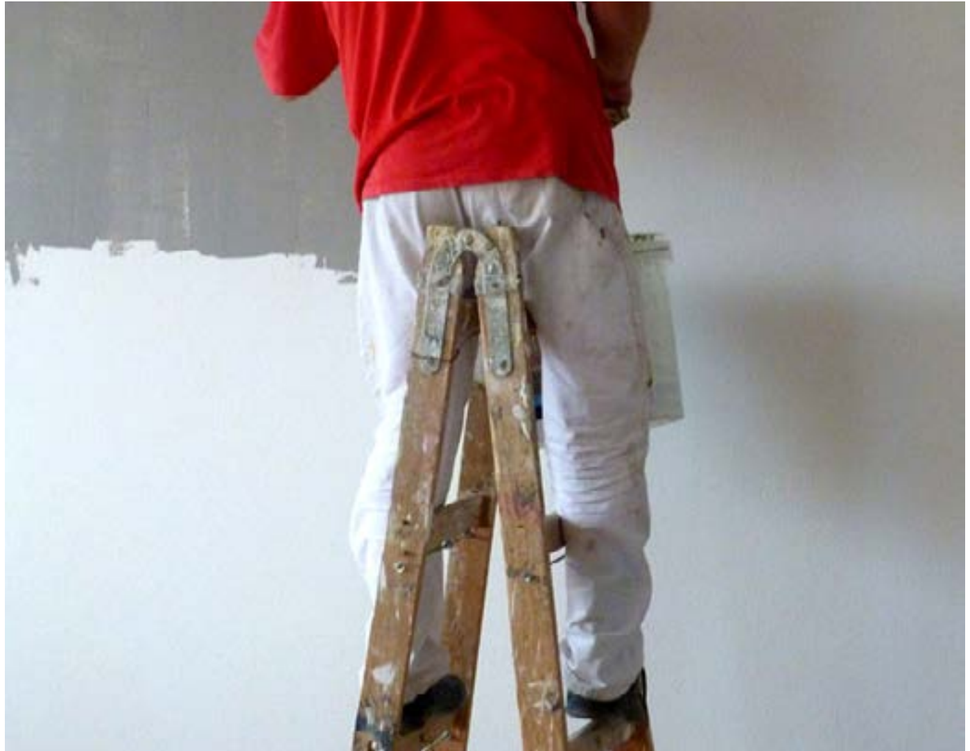
Fig: Applying the base coat, and leaving it to dry.
