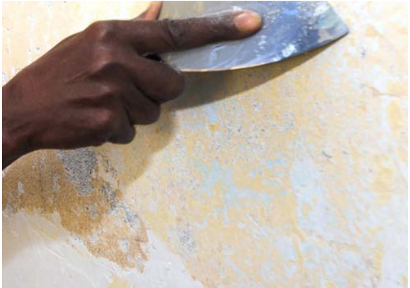
Fig: After scraping and filling the wall with cement putty, this is how the wall has to be evened out.
