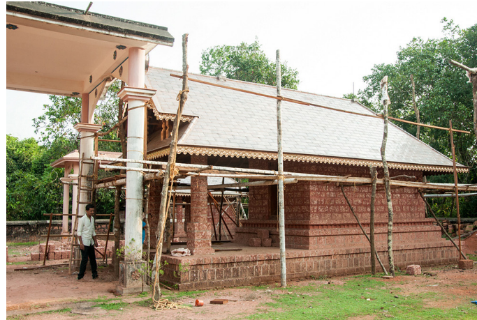
Structure of the Village shrine (Bhoothalaya) that is under construction.
