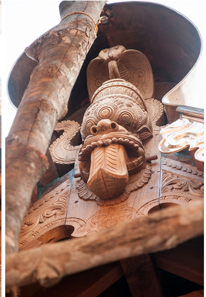
The close up of the roof from the exterior.
