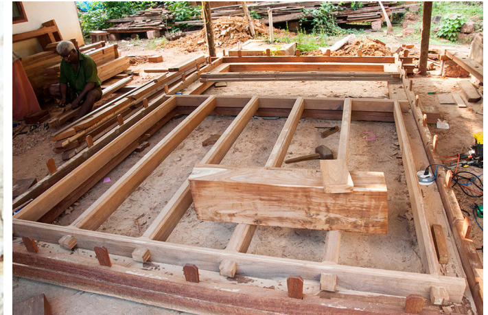
Further foundation of the roof is made at Bhoothalaya's sanctum.
