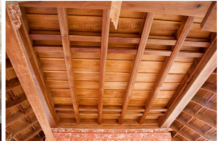
This wooden foundation of the roof is then fixed at the top of Bhoothalaya.
