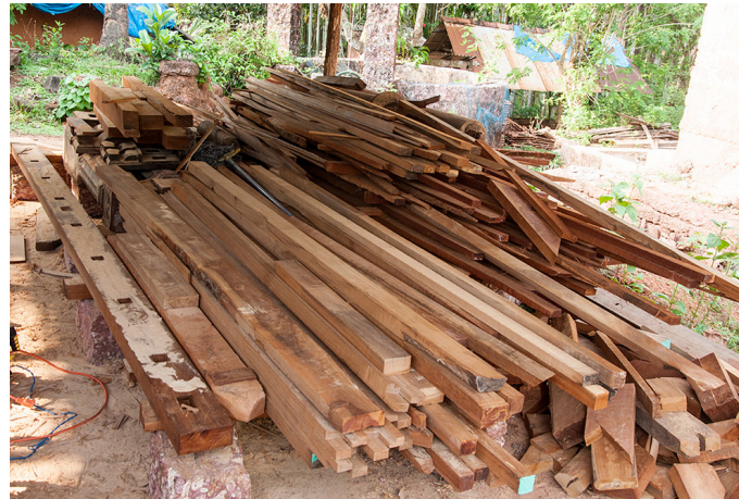
Wooden logs are cut and accumulated for the construction.
