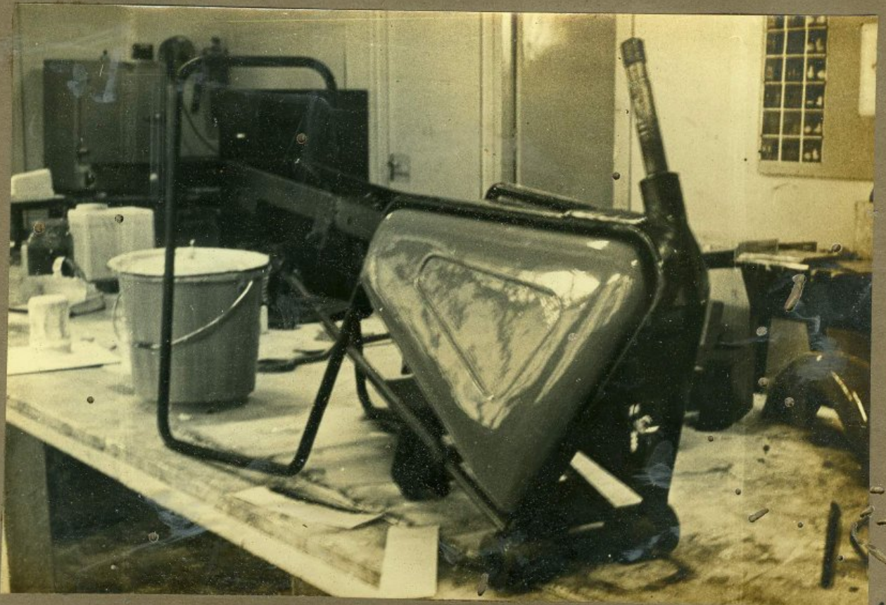
THE FRAME AT THE FABRICATION STAGE . THE TANK HAS BEEN FITTED FROM SIDE. 4
