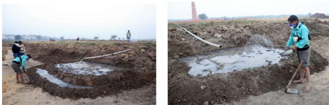
Figure 5-5: Pouring water into the soil (Left), Sprinkling salt to the soil (Right)
