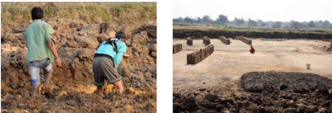
Figure 5-7: Stomping by feet (Left), The final mud (Right)
