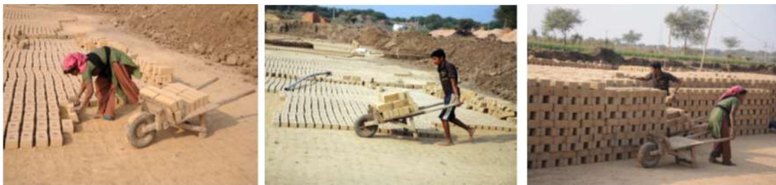
Figure 5-10: Stacking of bricks after moulding
