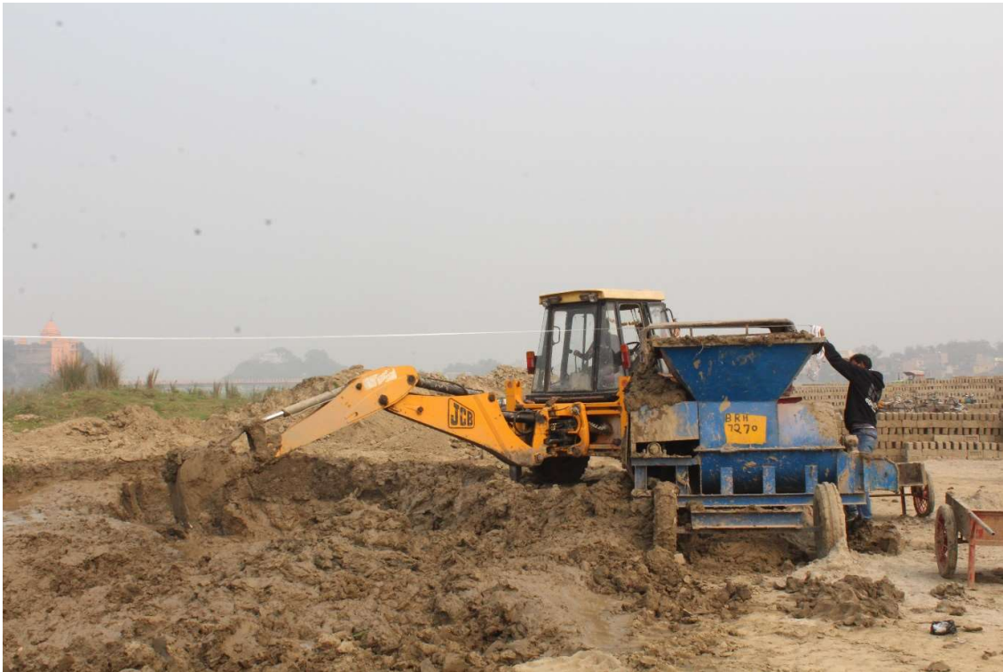
Figure 6-2: Mud mixing technique in SUN brick kiln industry, Bihar, India
