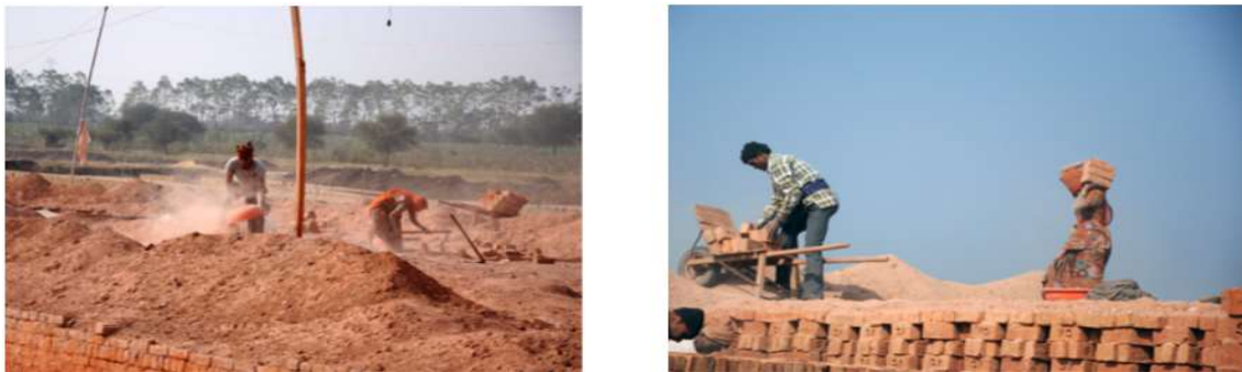
Figure 5-15: Removal of brick dust from kiln top
