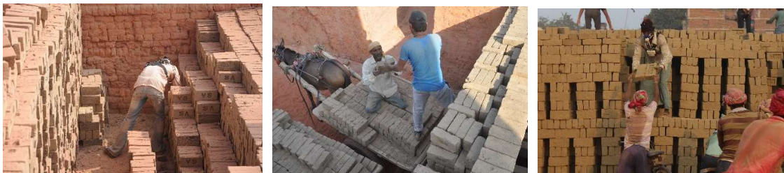
Figure 6-5: Khadkan's work method in the different studied brick kiln (Khadkan Bending in VS, Hand to hand transfer in RB and SUN)
