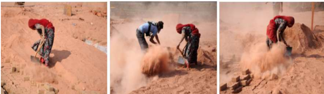
Figure 5-13: Covering the top part of the brick kiln by red brick dust activity
