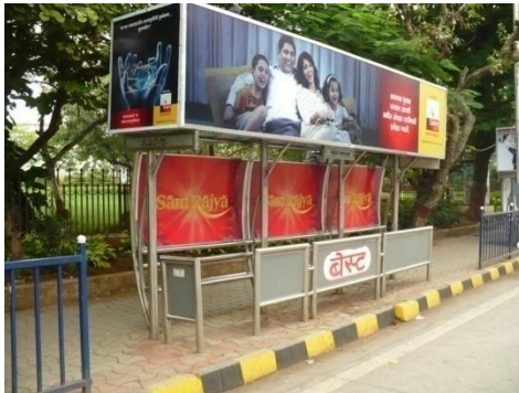
Fig. 4. Bus stop with shelter
