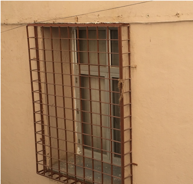
Fig 18: Grill fixed as a cantilever in one of the building inside IIT Bombay
