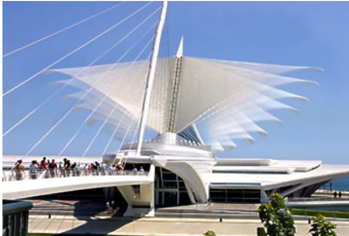
Santiago Calatrava, Milwaukee, Wisconsin, USA Spectacular kinetic structure Brise soleil with louvers that open and close like that of a bird.
