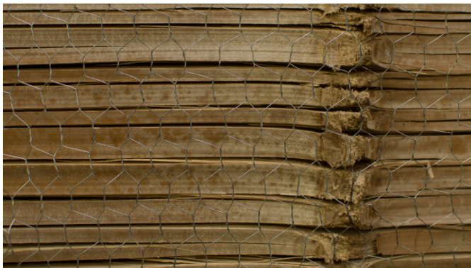
Fig.38: Wall construction using chicken mesh & bamboo
