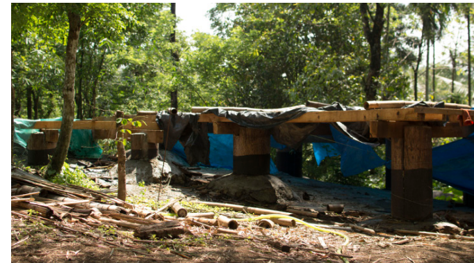
Fig.40: Palm and concrete base for construction
