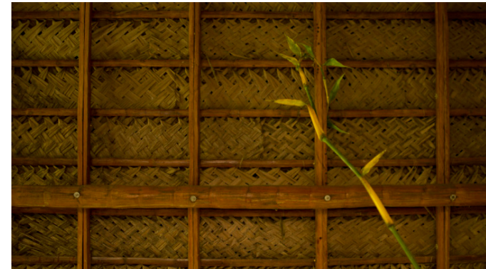
Fig.39: Roofing at Ecolinks
