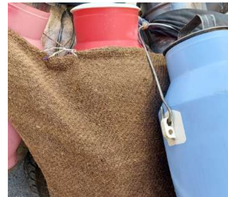
Securing secondary equipment - Raincoat, Wet jute cloth etc.
