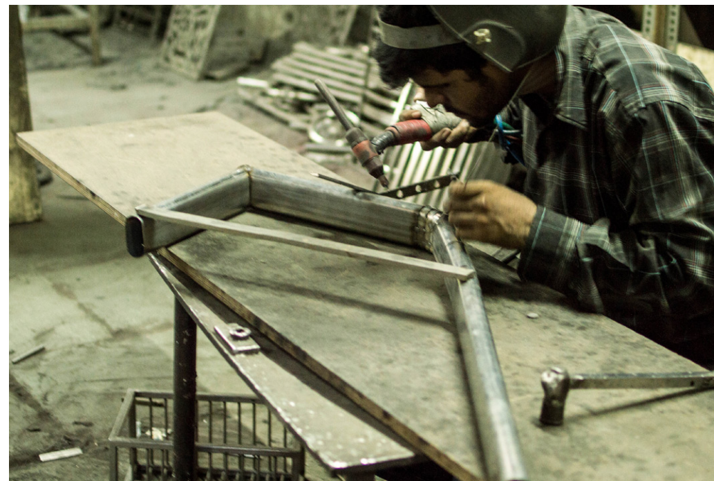
■ Welding the bends
