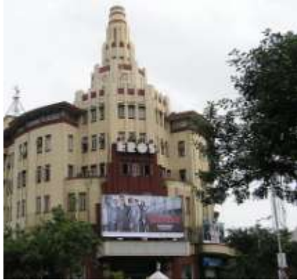
Figure 7.20 Eros, Bombay, built in 1938 Closest to exemplar
