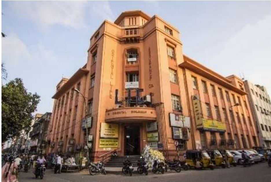
Figure 7.10 Oriental Building, Chennai, built in 1935
