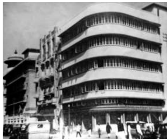
Figure 7.15 Kent House, Pheroze Shah Mehta Road, built in 1935
