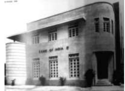
Figure 7.25 Bank of India, Bombay, built in 1938
