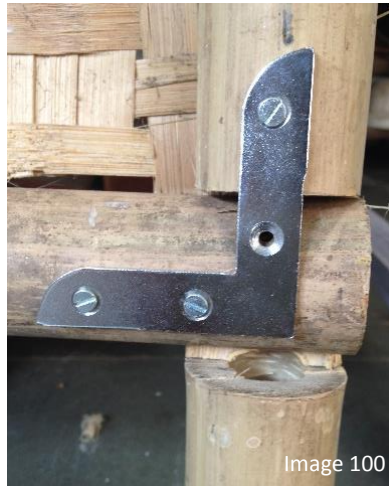
Two poles are fixed using a L joint
