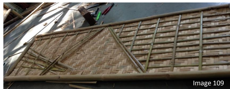
Bamboo panel (outside view) ready to be fixed
