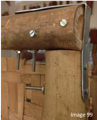
Two poles are fixed using a right angle
