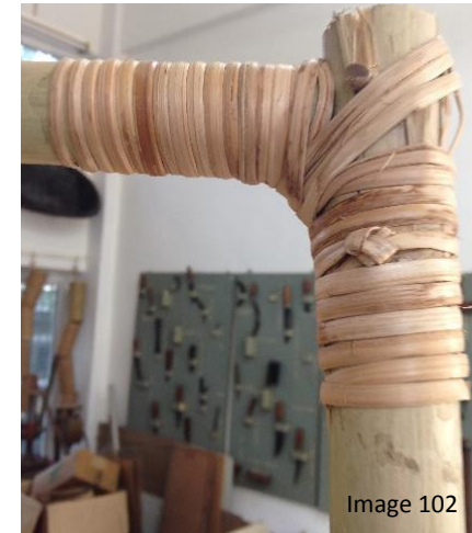
Two poles are tied together using cane
