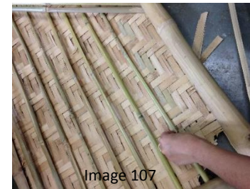
Bamboo strips are being attached to the mat to strengthen the structure which also adds to the aesthetic beauty of the structure
