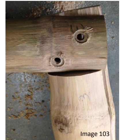
Two poles are fixed using bamboo nails.
