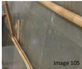
Slit bamboos joined together to make the frame
