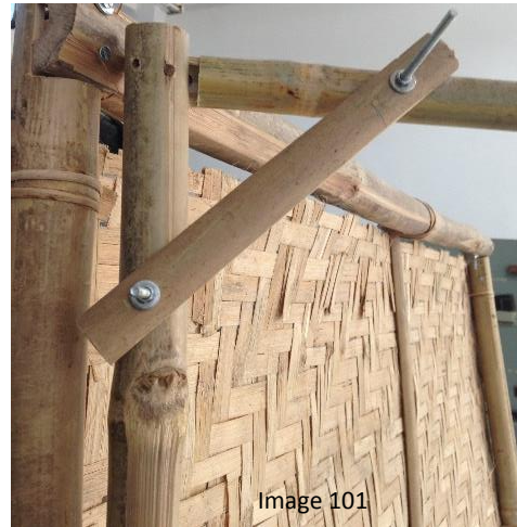
Two poles are fixed using a cross bamboo support with the help of nuts and bolt
