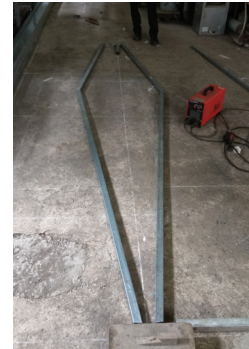
MS box members laid out during initial stage
