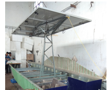
Panels are mounted and bolted
