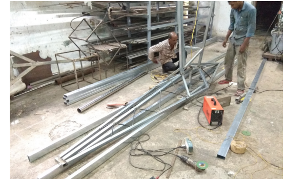
Finishing touches being made to the truss before inverting it
