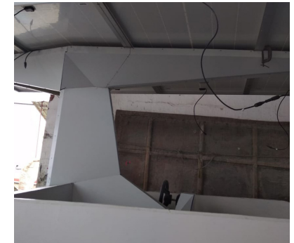
Panelling on the truss work
