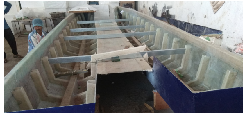
Hull pieces connected and steel beams are introduced
