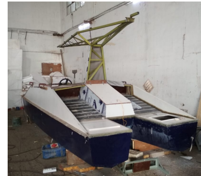
Battery box panelling using ACP
