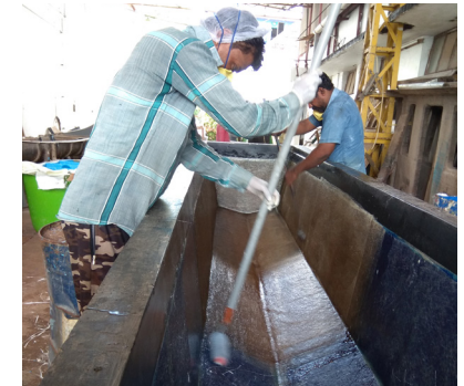
Resin applied onto the fibre using rollers
