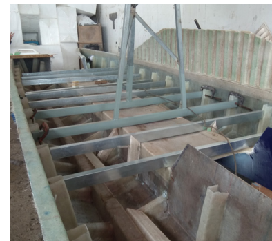
The truss legs are welded to the MS beams for support
