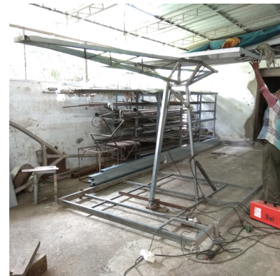
Solar panels being mounted on the erected truss system
