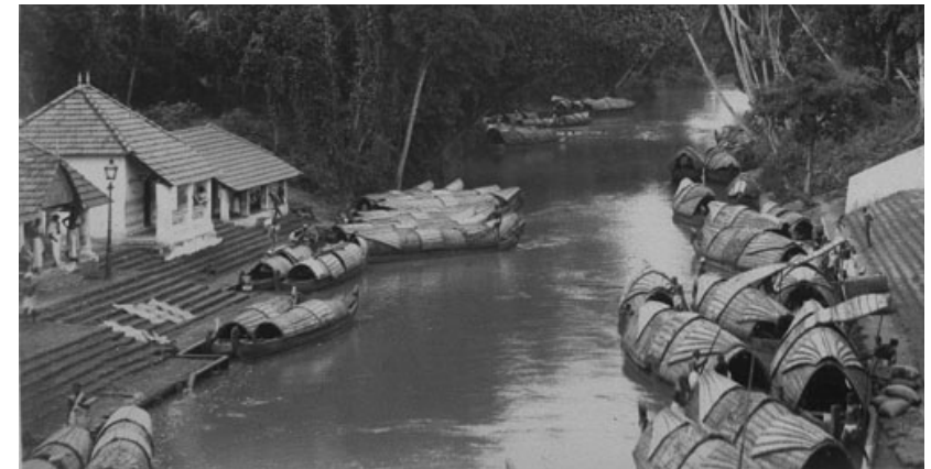
Img 20. Kevuvallams transformed into houseboats being docked in waterways
