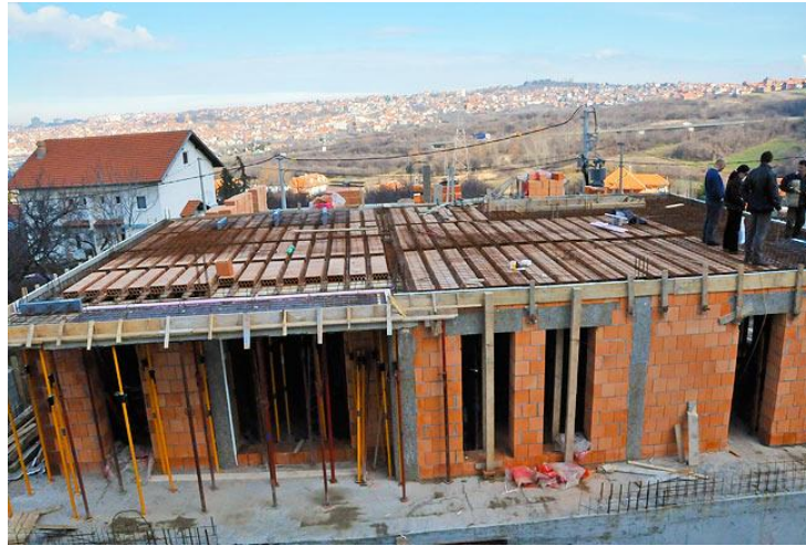
Fig. 3: A typical under-construction house http://beodom.com/sr/news/entries/amadeo-2-1st-floor-slab-and-installation-of-avi-thermokorb as seen on 12/11/2014
