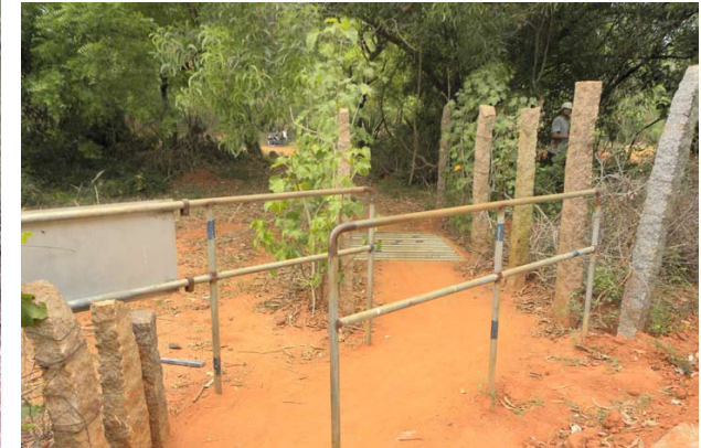
The cyclists have to get down while going through the motorcycle barrier. this causes inconvenience.
