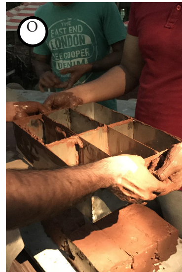
Using two persons to lift the mould
