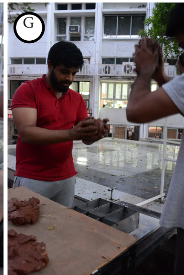
Throwing the mud into mould
