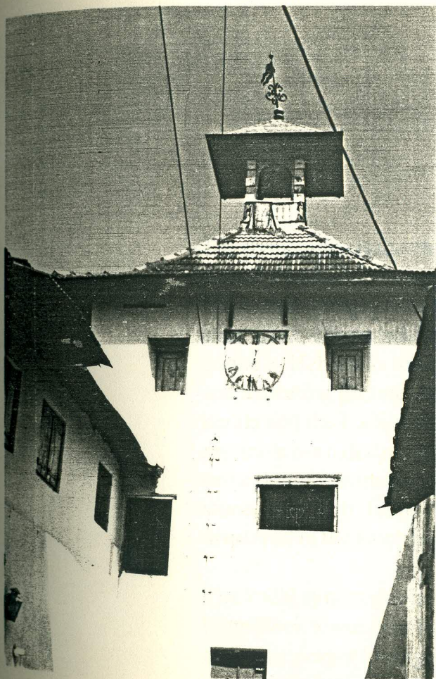
THE CLOCK TOWER OF THE CHURCH
