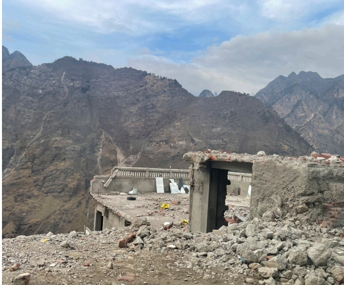
Fig 2.8 Issac, R., A concrete structure that was demolished, one among many. Joshimath. 2023.
