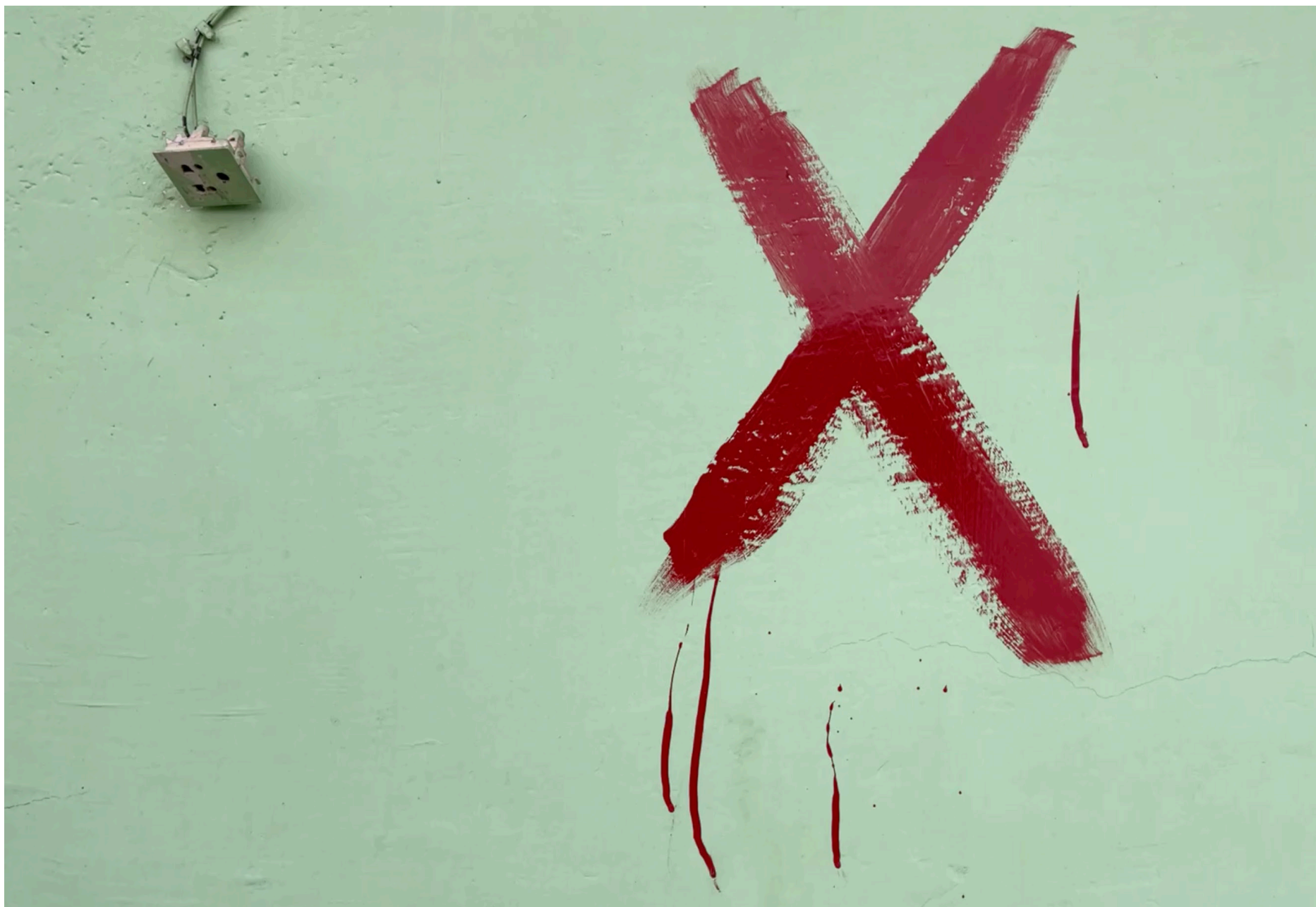
Fig 2.5 Issac, R., House to be demolished marked with an 'X'. Joshimath. 2023.
