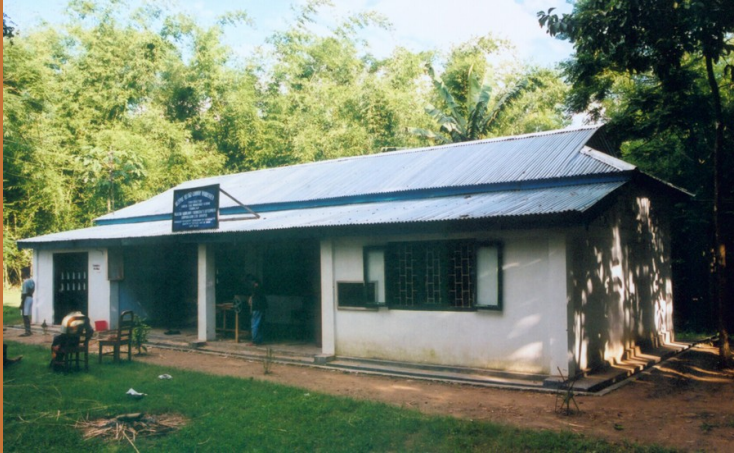
CFC - work shed
