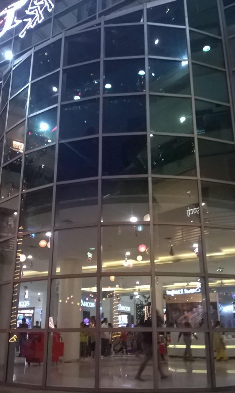
Front glass facade
